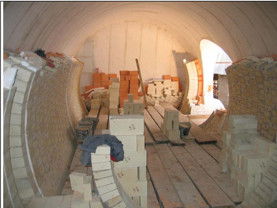
Refractory Lining in a Sulfur-Burner
