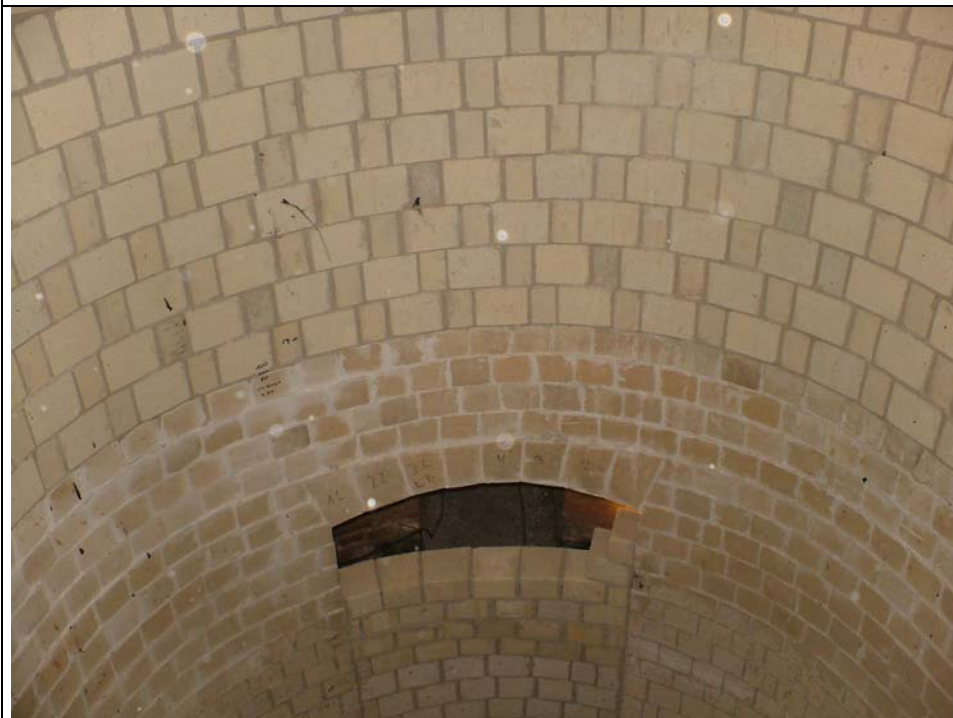
Relining of a chimney
